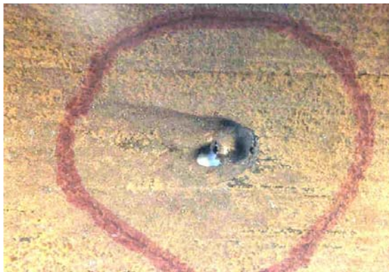
Figure 3 Erosion-corrosion Around Deposits (Photo Courtesy of Howell Image Sciences)
